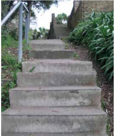
Photo 13. DDA compliant access is not catered in the existing condition
